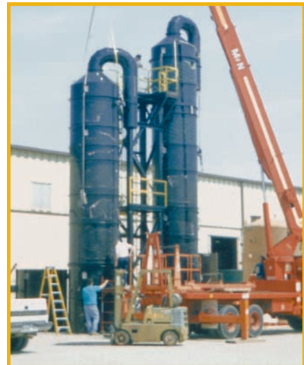
Application: Specialty steel production (acid etching) Problem: NO x and mixed acid fumes Solution: Beta NO x 2000® Two Stage
